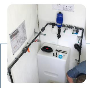
Design and supply of a **Gravikit 3D25** for a disinfection of a military source in Piène Haute France
